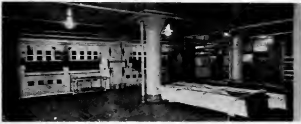
VIEW IN BAKERY DEPARTMENT ON SECOND FLOOR
